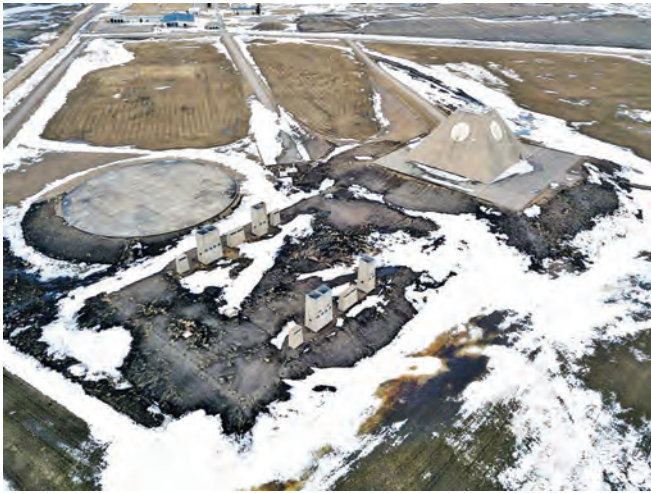
Drone photo of the bunkers. MSCB with the turret in the background, MSPP in the foreground with the heatsink upper left. Photo Chris Howells
